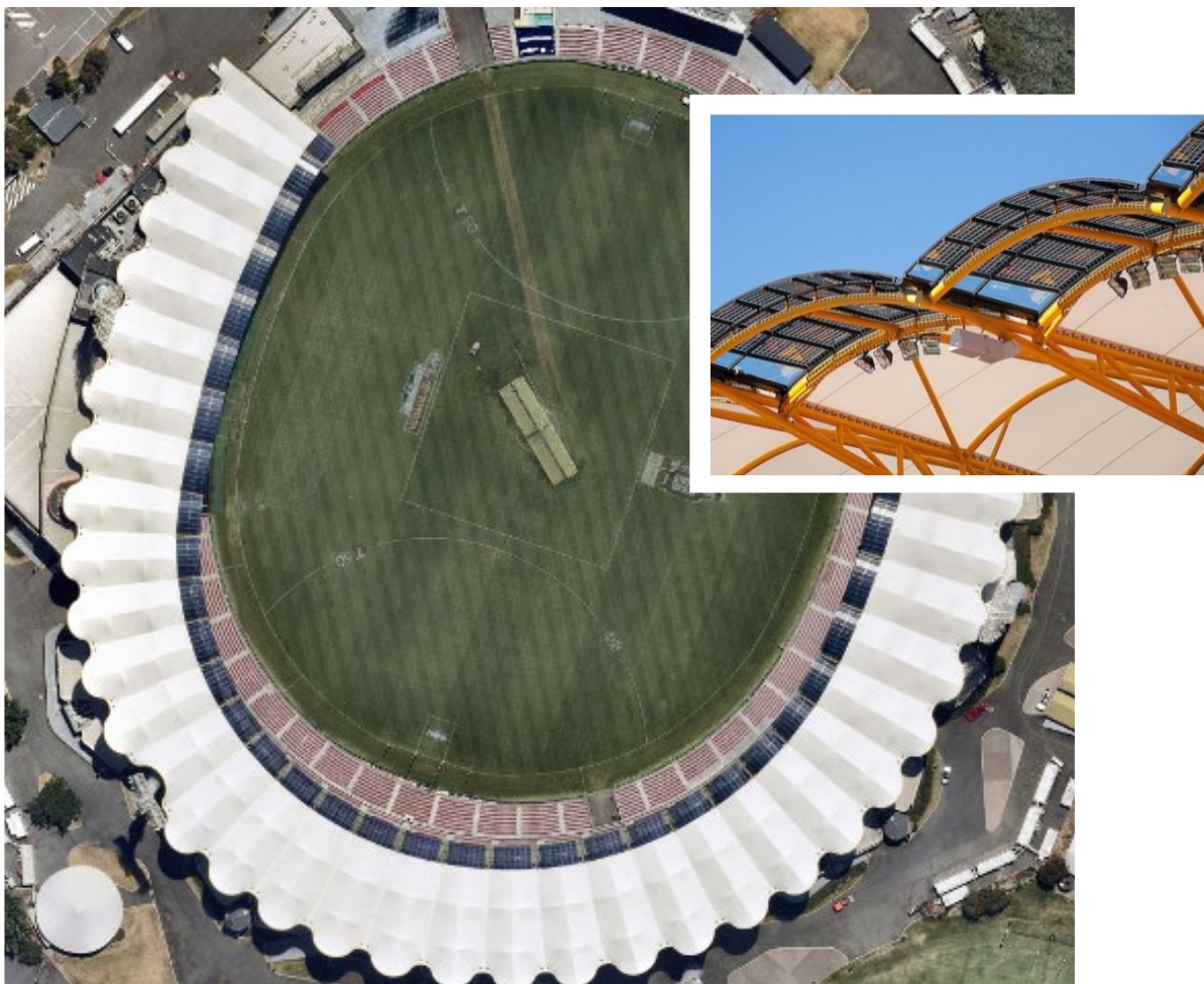
Figure 10: Existing 200 kW “solar halo” at Metricon stadium
